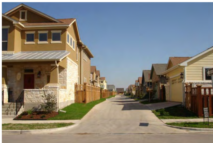
Figure 6: The alley provides these Austin, Texas homes with a zero-step entrance through the garage.
